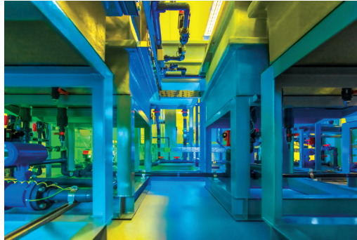
FIGURE 5: RESERVOIR TANKS AT DIFFERENT STAGES OF THE WADI TESTBED
